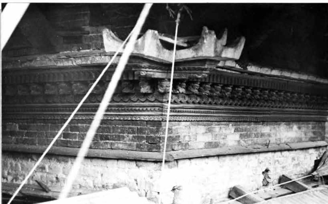
Upper level of rooftop pagoda shows dacia apa framed by timber cornice pieces. Below common fired brick with visible mud mortar joints. All in excellent condition.
