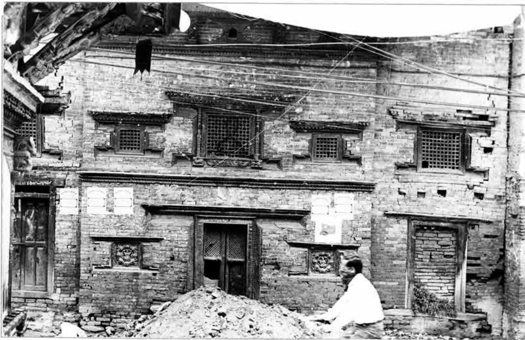
Front facade, lower two stories. April 1993
