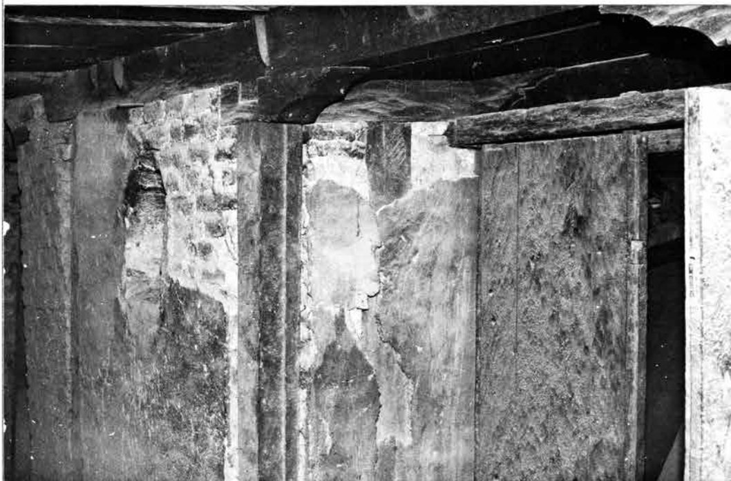
Three pairs of timber columns in front of esoteric shrine, second floor. Summer 1993.
