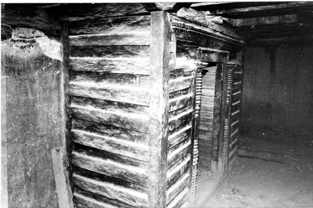
Timber partitioned esoteric shrine, second floor.
