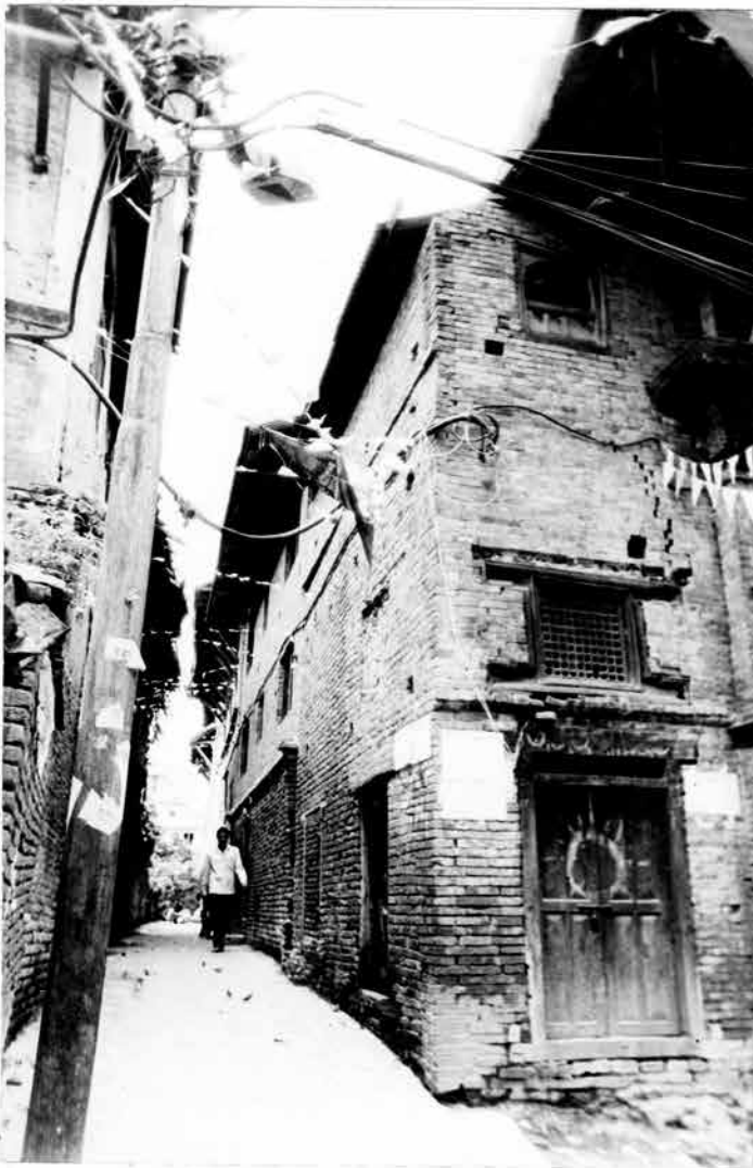
Southeast corner: notice later patch at corner at plinth level. August, 1993.
